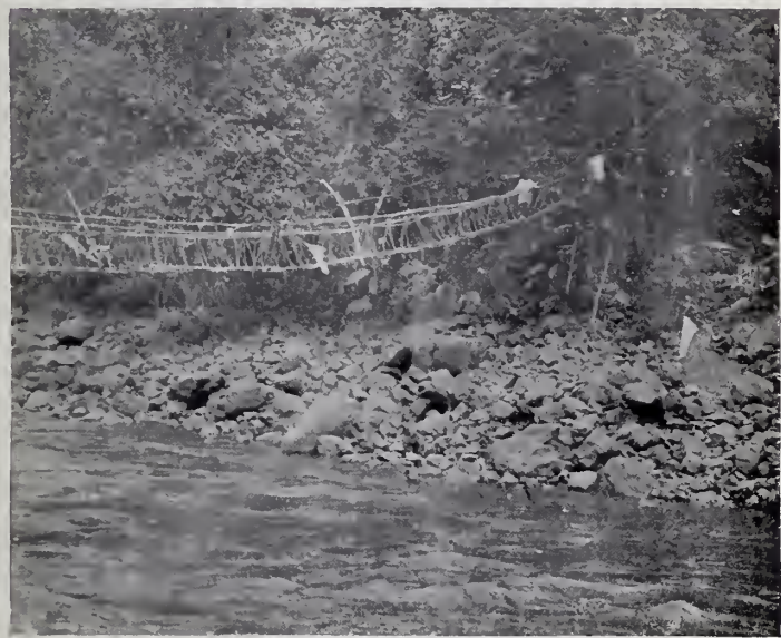
1.—LOOKING DOWN A NATIVE HANGING BRIDGE.
